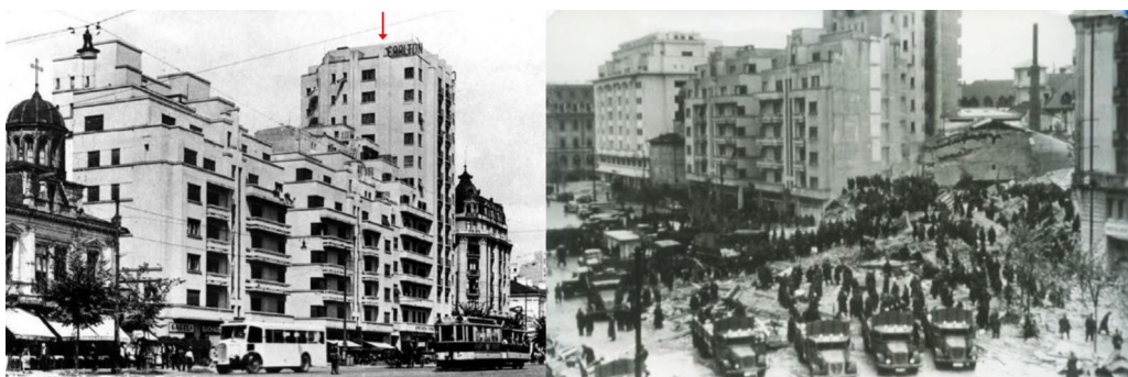
Figure 6.5 Carlton building in central Bucharest: before and after the 1940 earthquake. The building had been finished only 4 years before the earthquake
