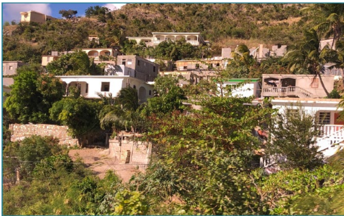
Figure 5.8 Housing construction on hilly terrains. Source: World Bank (2020,p.38 ) Rapid Housing Sector Assessment: Sint Maarten
