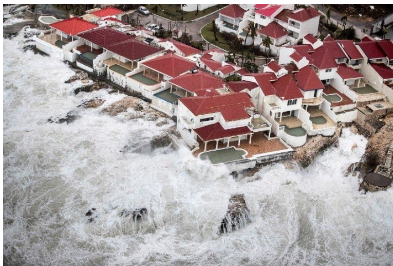
Figure 5.6 Coastal erosion due to Hurricane Irma. Image source: https://nltimes.nl/2017/09/07/videos-hurricane-irma-leaves-trail-destruction-sint-maarten-saba-sint-eustatius
