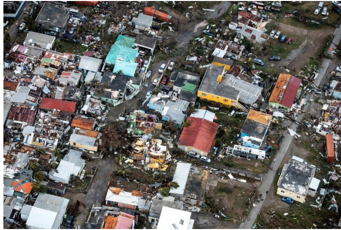
Figure 5.4 Physical damage caused by Hurricane Irma. Source: An aerial photograph taken by the Dutch Ministry of Defense shows the devastation caused by Hurricane Irma in Philipsburg, on the Dutch Caribbean island of Sint Maarten, Photo Date: 9/7/17 (WHSV):
