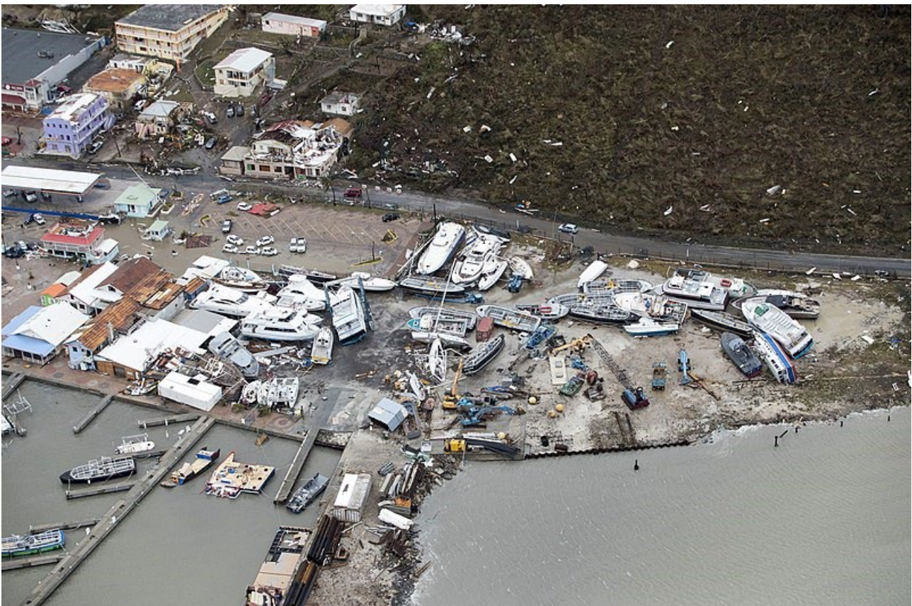
Figure 5.5 Damage to the harbour caused by Hurricane Irma. Image source: https://commons.m.wikimedia.org/wiki/File:Alh-08-09-sint-maarten-foto-6-duo.jpg#mw-jump-to-license
