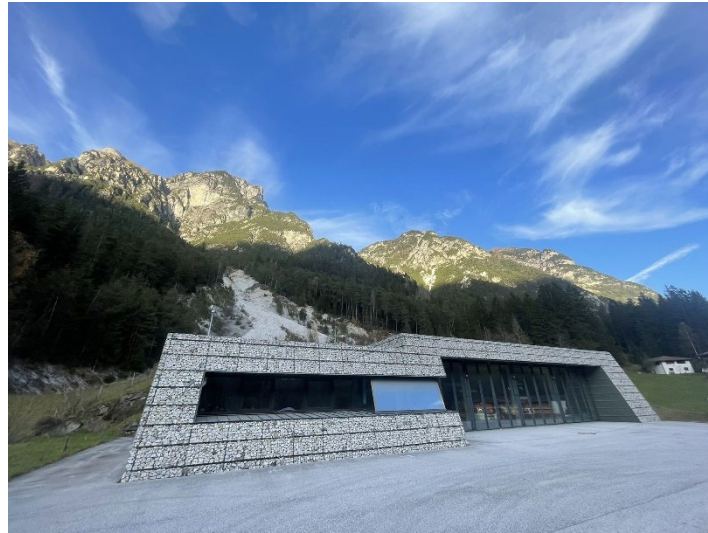
Figure 3.2.2: Protection measure in South Tyrol with a double use (Source: Andlinger, 2024).
