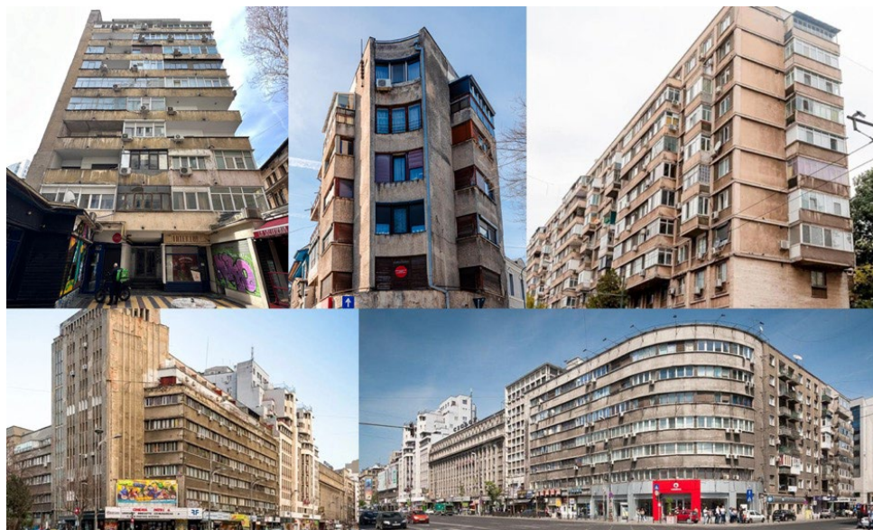
Figure 2 Selection of buildings planned for retrofitting in Bucharest
